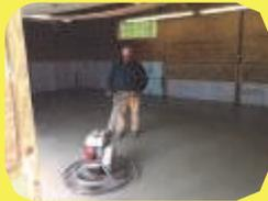
What a job! Thanks to help from Kenneth Gallion and Gallion Trucking and Excavating, we were able to dig out the rotten, water-logged floor of the woodshop (and the 2-3 feet of muck underneath) so that we could backfill it with gravel and then top it with concrete for a safe and sturdy floor that will last!
