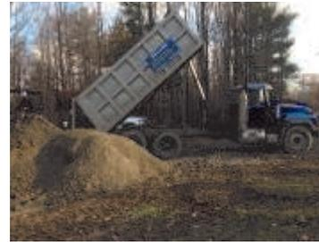
We are thankful for Gallion Trucking and Excavating that supplied the trucking and Keeney Sandstone & Quarry that donated over 20 loads (400 tons) of backfill compaction sand for the Philippians Building. JEO Construction then provided the machine and John Ostyke (owner), operated the machine to put the compaction fill in the building.
