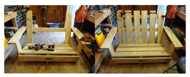
After the backs are mounted, use the remaining piece of the back support on the top of the boards. Cut ~6" off the length and clamp it in place while fastening. Flip the chair on its top, with the arm rest and top of the seat back touching the floor. Pre-drill and fasten the lower edge of the backs to the seat, using two screws a board. Take one of the scraps and cut 45° angle on one end. Fasten that piece to the side of the middle rear leg and the back board. (See picture)
