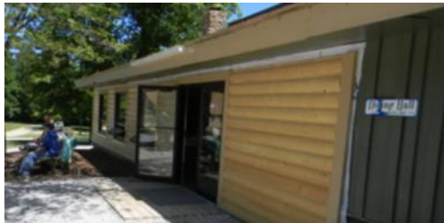
New wood siding and windows make it look and feel like a new building.
