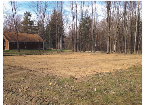
The cleared pad at the end of the day
