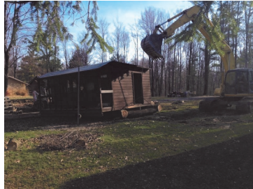
Getting ready to move the old store
